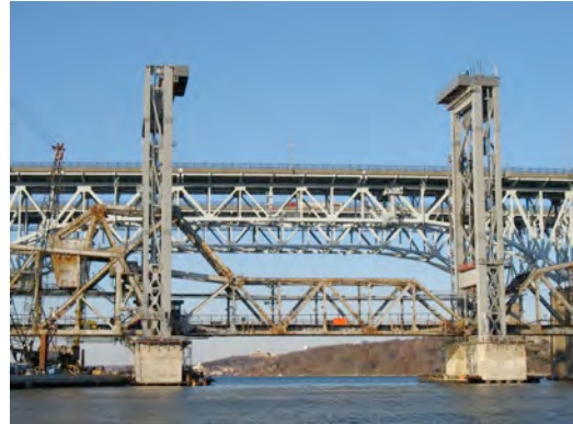
Figure 1: Existing bascule during construction of the new vertical lift towers.
