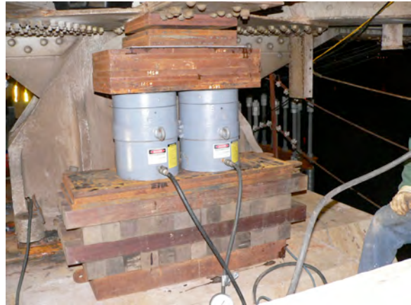
Figure 8: Two 430 ton capacity rams.
