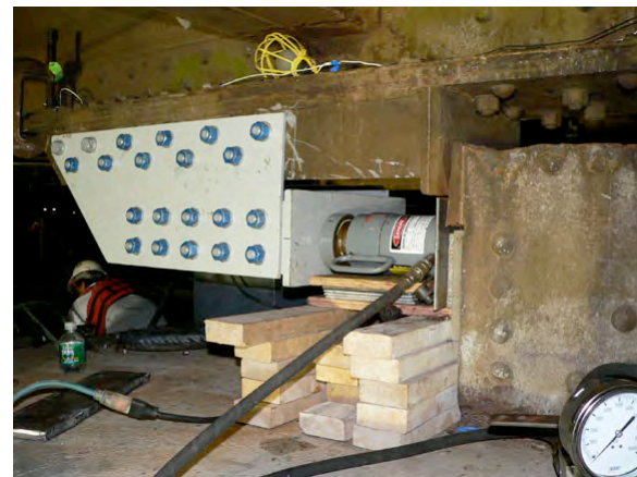
Figure 9: Lateral Jacking bracket.
