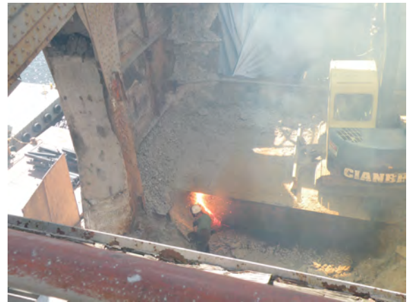
Figure 11: Cutting steel and concrete.
