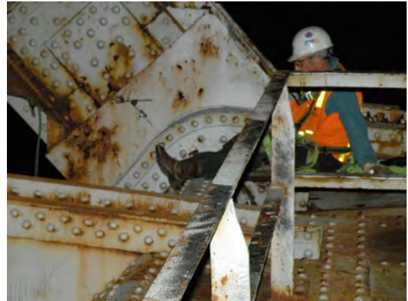
Figure 6: The lonely job of monitoring the counterweight link at the bascule span.
