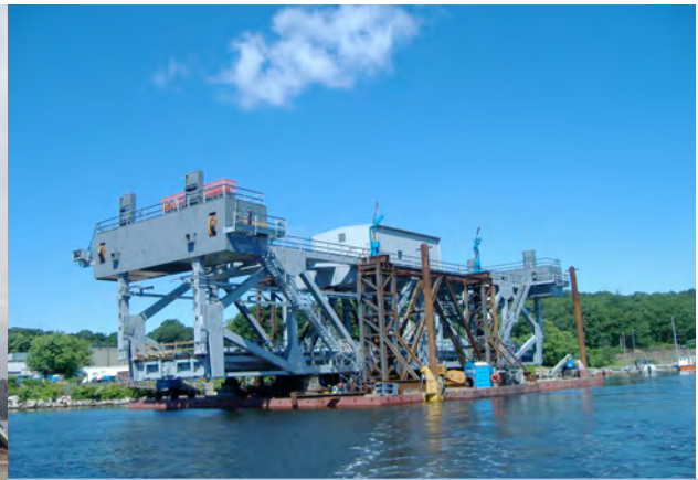
New lift span ready for float in
