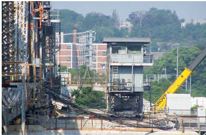
Control house after being moved on the pier.
