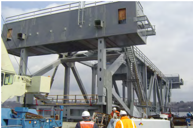
New lift span on barge near completion
