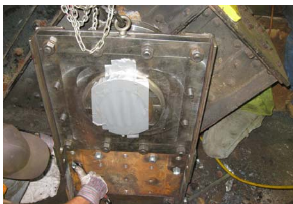
Figure 26 – Hanger assembly being splice into existing cast-in hangers
