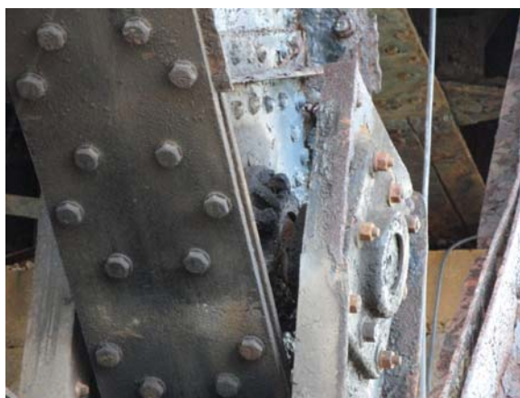
Figure 4 – Bent outboard hanger and sheared counterweight trunnion pin
