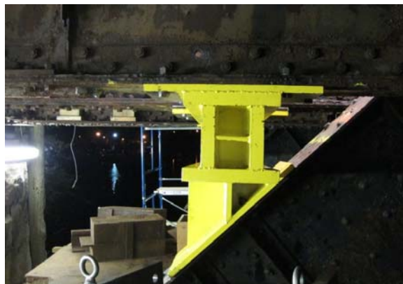
Figure 16 – Chock assembly engaging the bascule girder and approach girders
