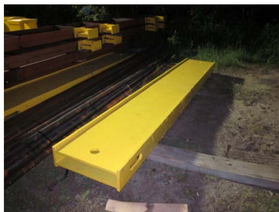
Figure 9 – Lifting beams in staging area on site
