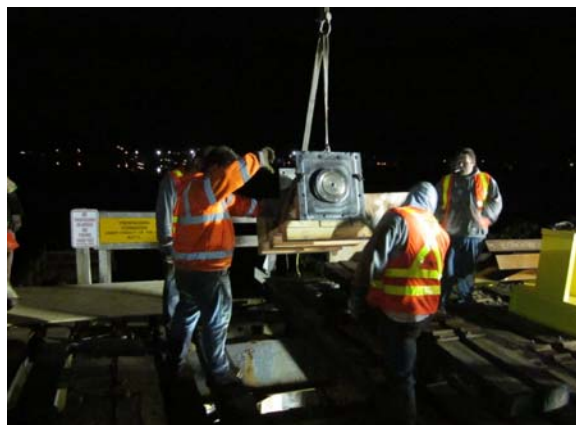
Figure 17 – Bearing assemblies being lowered to the counterweight
