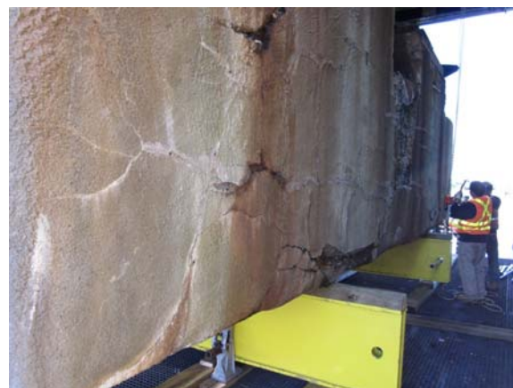
Figure 20 – Lifting beams being installed under the counterweight
