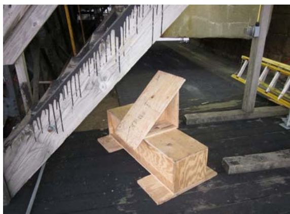
Figure 12 – Mock up chock assembly in the field
