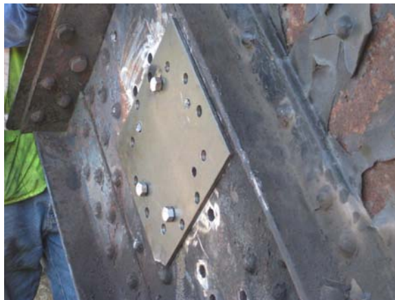
Figure 25 – Bolt template being used to drill the new bolt pattern into bascule girders
