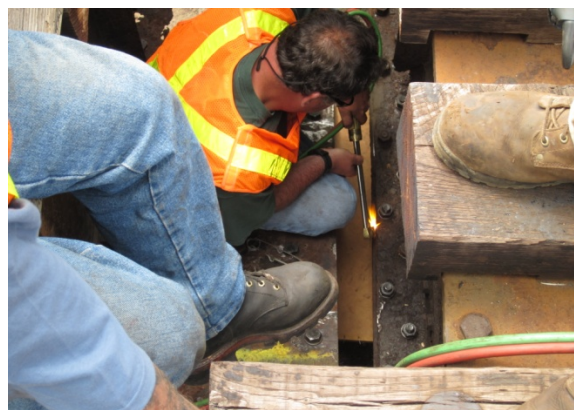
Figure 27 – Modifications to the approach span girders
