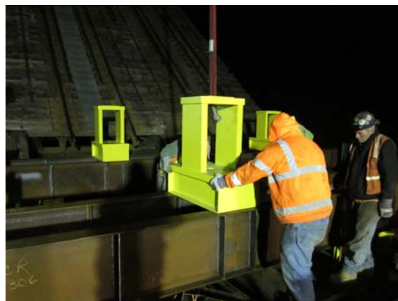
Figure 19 – Jacking seat being installed
