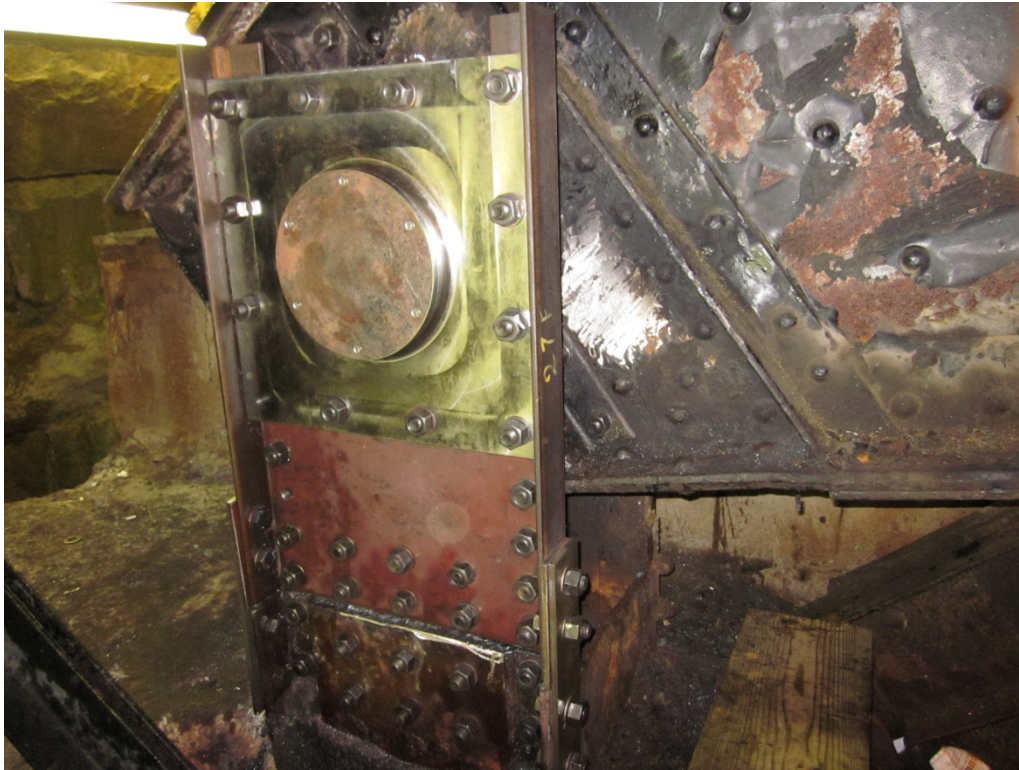
Figure 28 – Completed installation of counterweight trunnion pin
