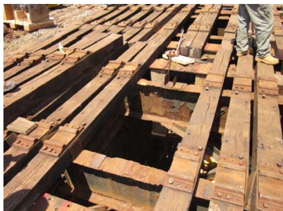
Figure 13 – Opening in the approach span to access the top of the counterweight
