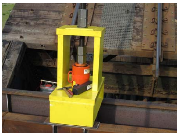
Figure 22 – Complete jacking assembly
