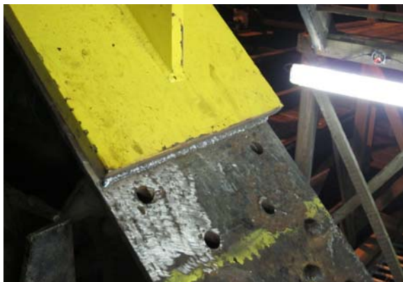
Figure 15 – Chock assembly engaging the bascule girder and approach
