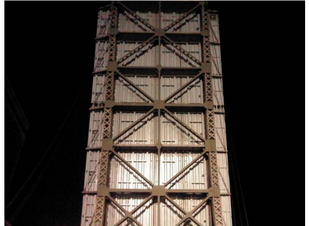
Underside of orthotropic deck in the open position
