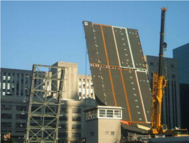
Orthotropic deck during erection
