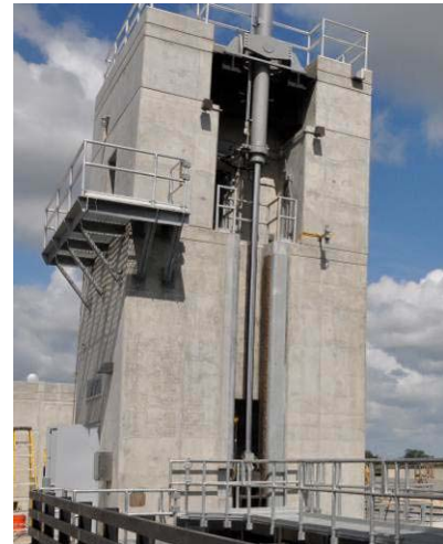
One of four 23' stroke hydraulic cylinders that lift the vertical lift gates
