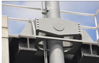
Cylinder Cardanic Ring Assembly
