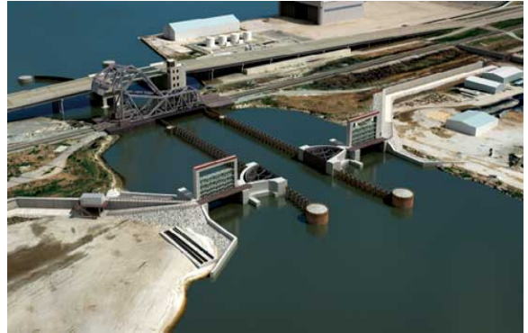
Overhead view of sector and lift gates at Seabrook Gate Complex
