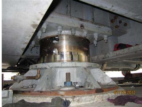
Photo 2: New Center Bearing (Oil box and dust skirt removed)
