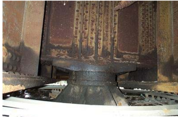
Photo 1: Existing Center Bearing
