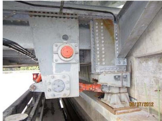
Photo 11: New end wedge machinery (outboard side)
