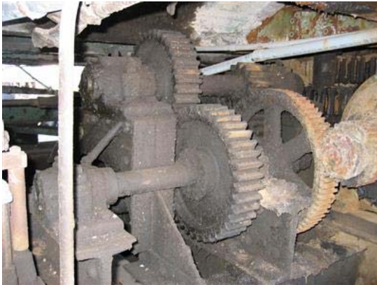
Photo 6: Original span drive gearing
