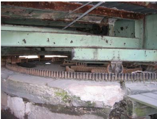
Photo 8: Original Rack and Balance Wheel and Track
