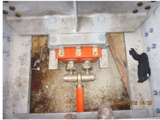
Photo 13: Top view of new center wedge.
