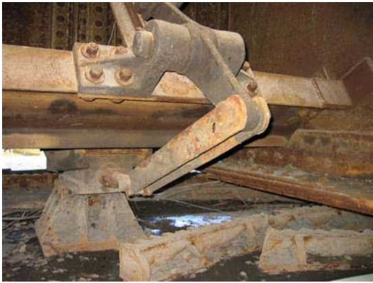
Photo 12: Original Center Wedge and Center Wedge Machinery.
