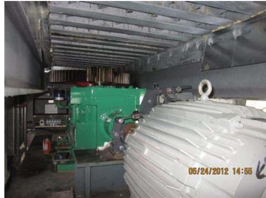
Photo 7: Redesigned Span Drive Machinery
