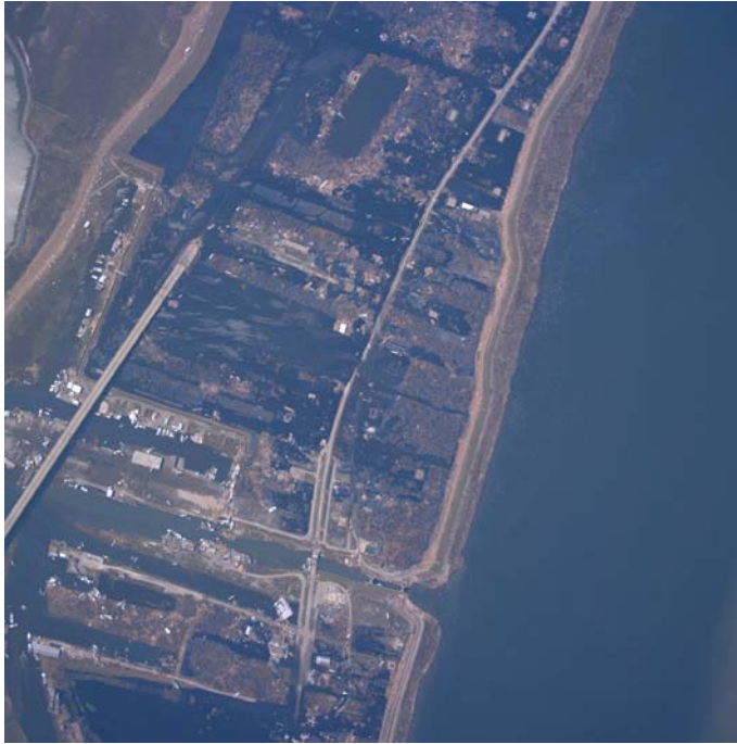
Figure 4 - Doullut Canal after Hurricane Katrina
