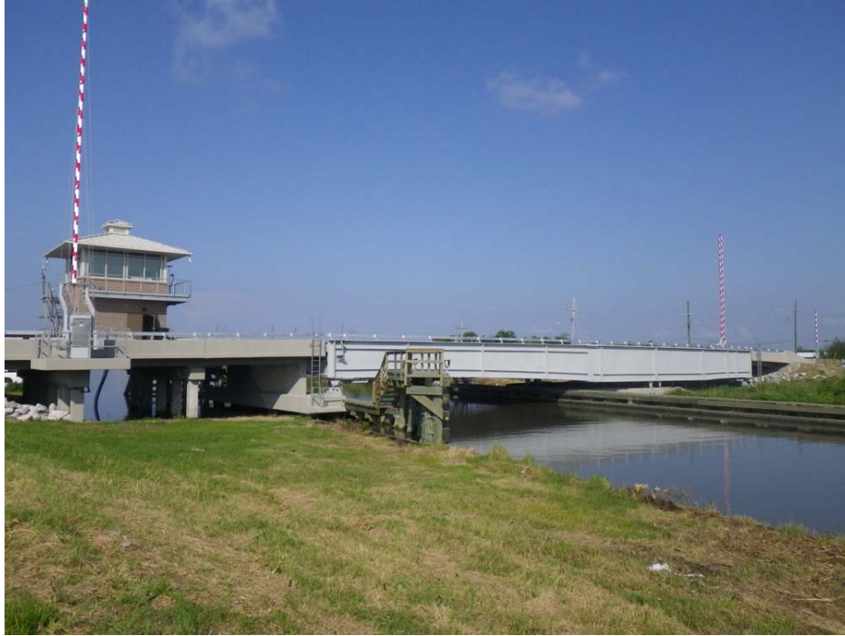
Figure 3 - New Doullut Canal Bridge
