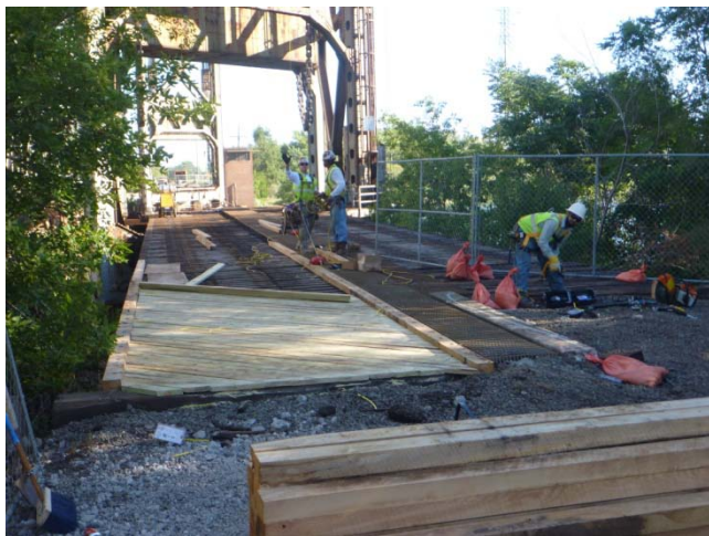
Installation of timber roadway decking on existing ties, approach spans
