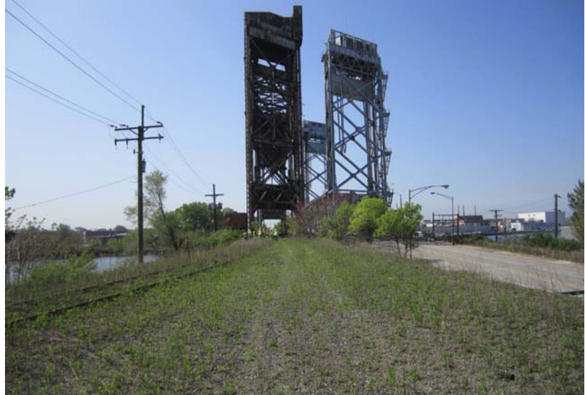
C&WI Bridge (left along abandoned track) and CDOT Torrence Avenue Bridge (right) looking south
