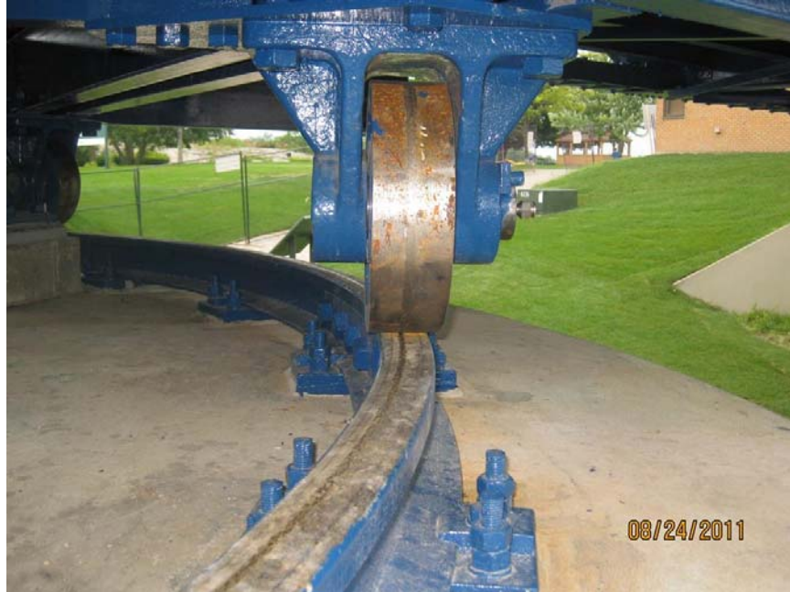
Photo 2: Balance Wheel and Rail
