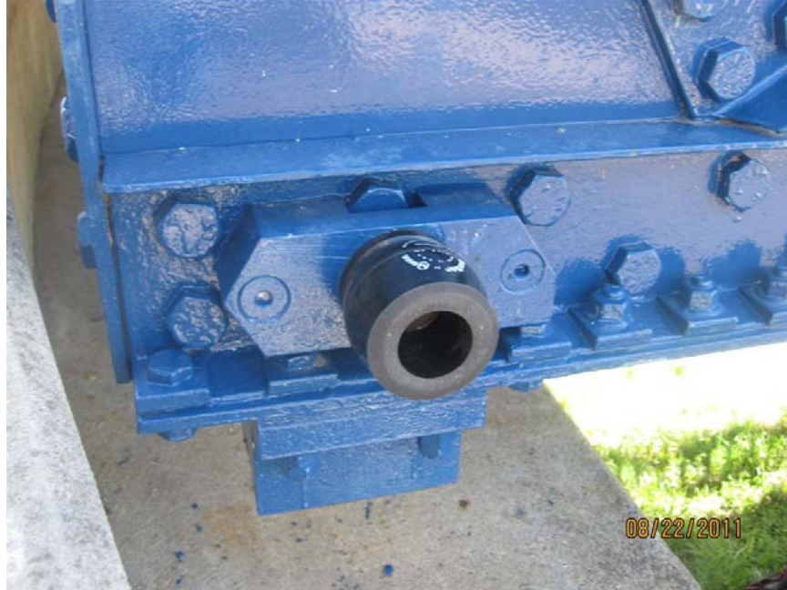
Photo 6: Energy Absorbing Bumper Mounted to the Span
