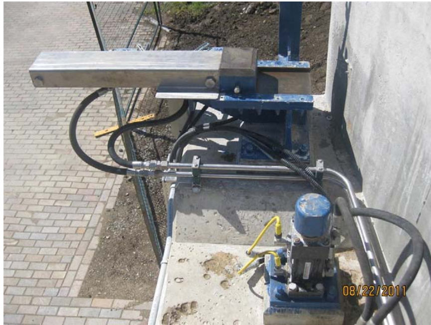
Photo 3: New Installation of the End Jack and End Wedge
