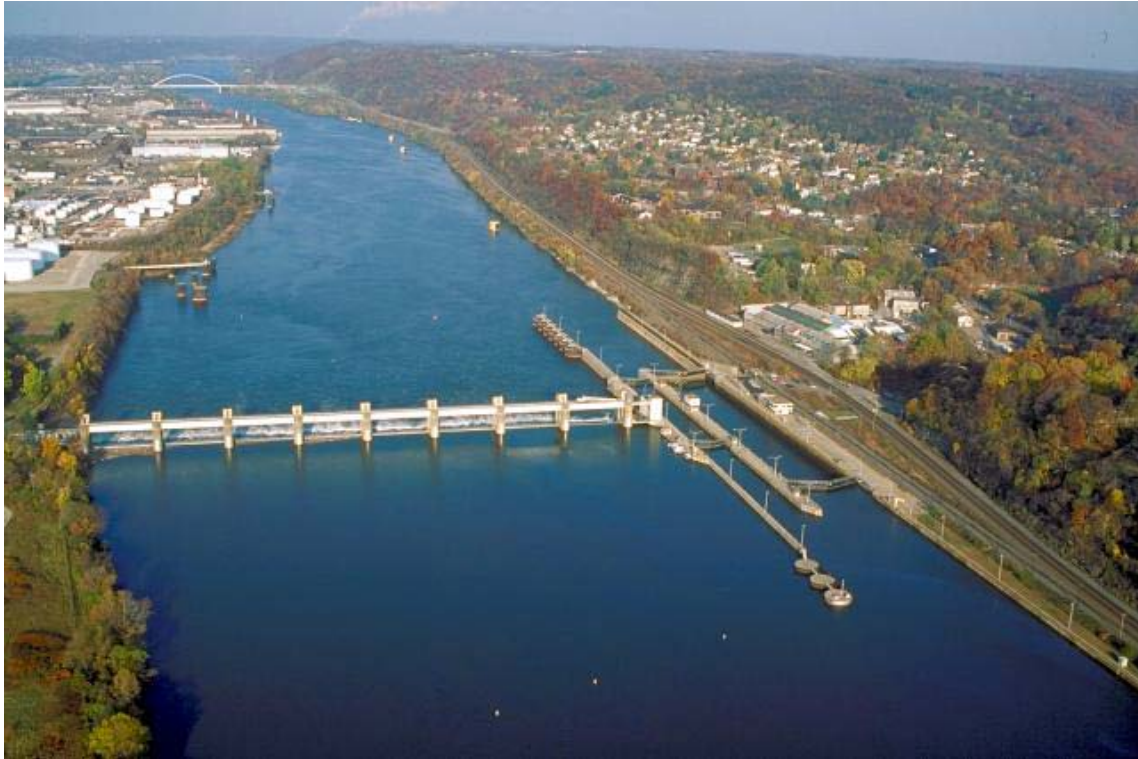
Figure 2. Emsworth Lock and Dam Main Channel
