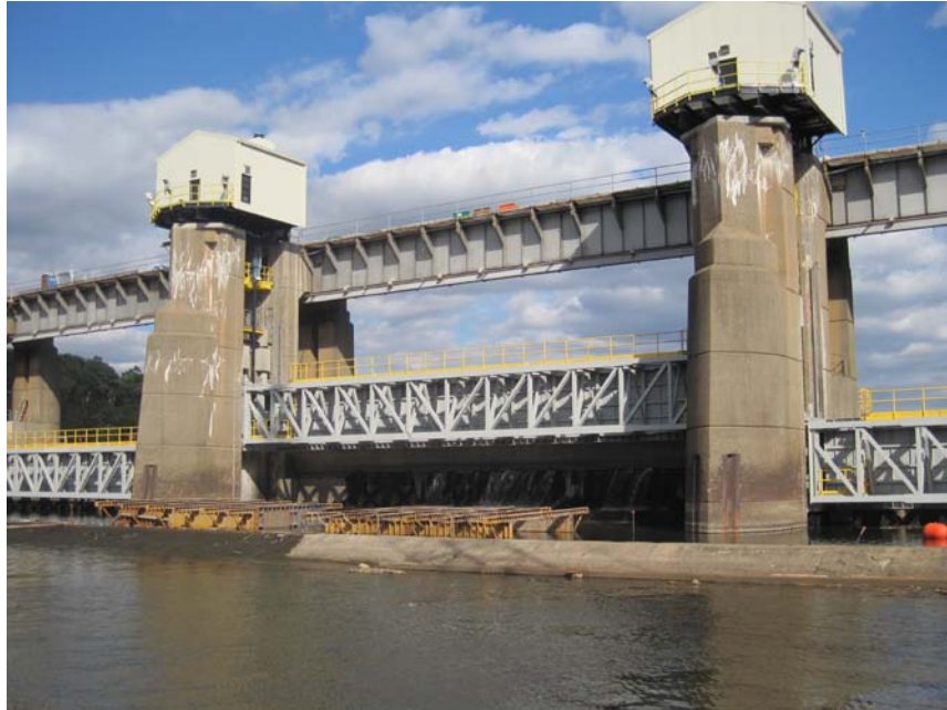
Figure 3. Spillway gate
