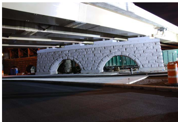
FIGURE 15: Arched Granite Faced Piers
