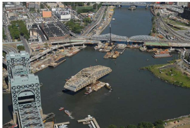
FIGURE 7: Swing Span Float in Operation
