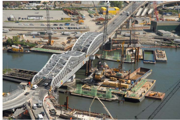
FIGURE 6: Off Line Pivot Pier Construction
