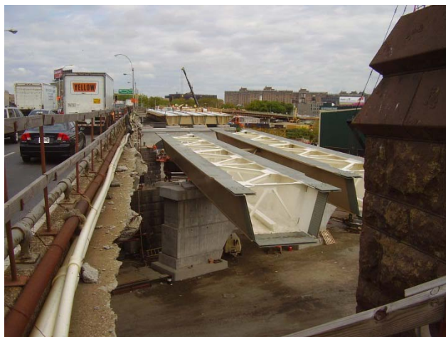
FIGURE 14: Trapezoidal Box Girder Spans
