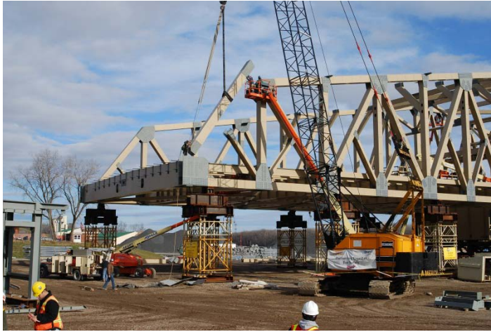
FIGURE 18: Truss Assembly near Albany, NY
