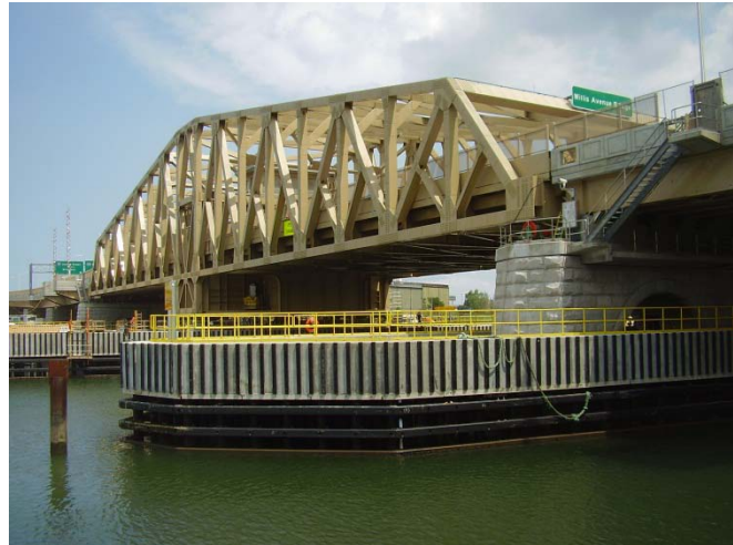
FIGURE 20: Fiber Reinforced Plastic Fender System
