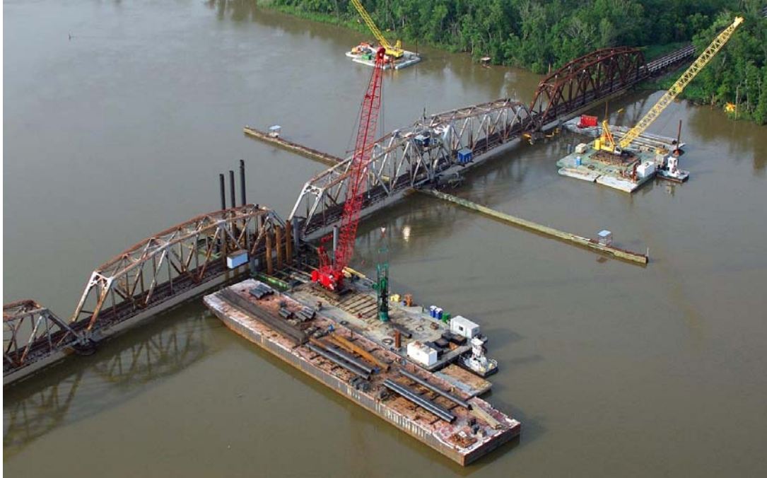
FIGURE 6: Bridge during construction, with piles driven at Pier 2B.
