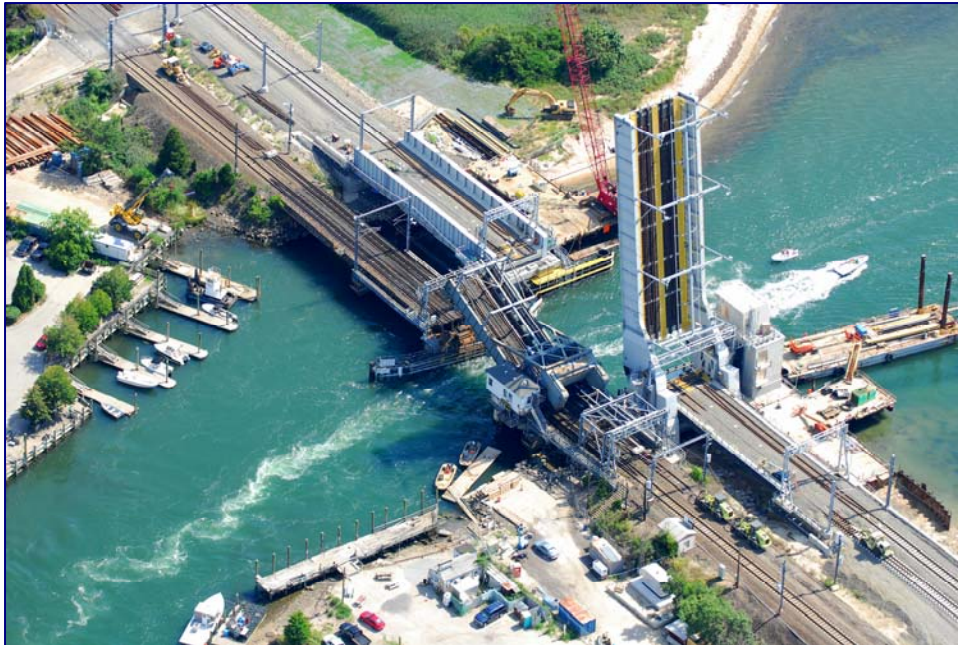
Figure 8: August 25, 2012 Two weeks before Placing the New Bridge in Service
