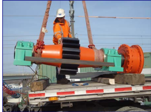
Figure 3: Bridge Drive Pinion Delivered to Bridge Site
