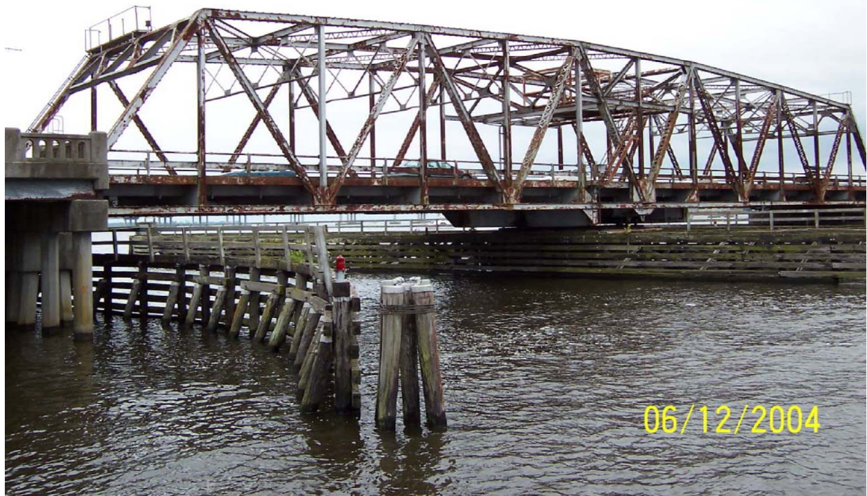
Figure 1. Elevation of Existing Swing Span of Bridge
