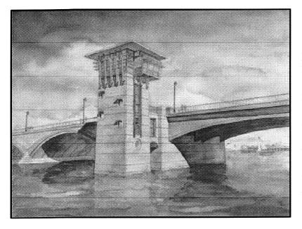
For the bascule span the conditions established by the Landmarks Preservation Commission had two principal impacts. First, the requirement to feature the arch form was carried through the bascule span. This was incorporated into the design through the use of an exaggerated variable depth of the bascule main girders. Furthermore, the bascule span was configured with a small deck overhang, in other
