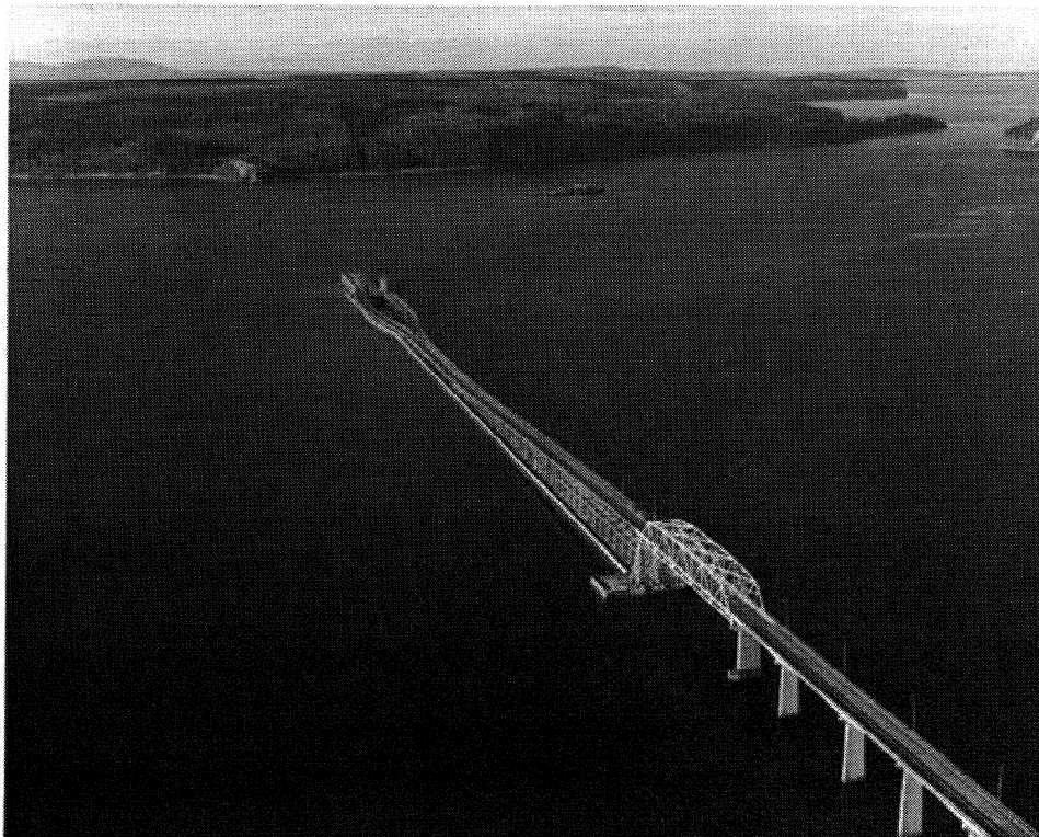
Photograph 8: Hood Canal Bridge with West half missing. 1979.
