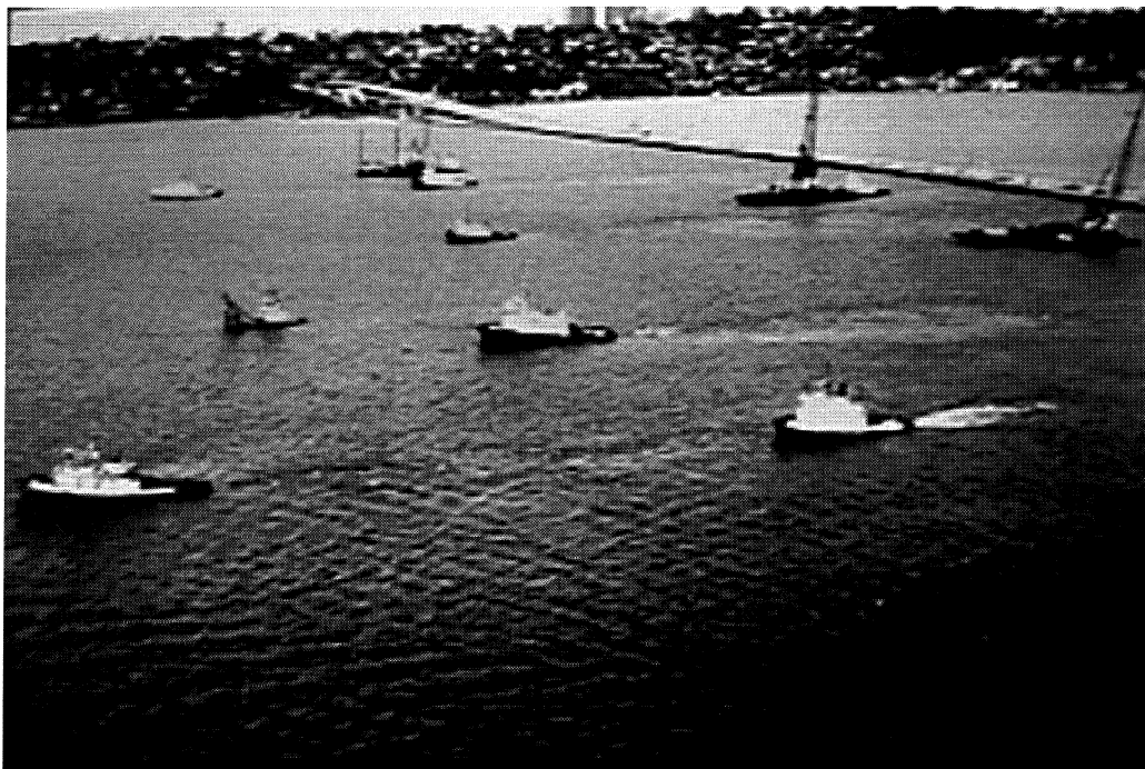
Photograph 4: Tugboats holding the new Homer Hadley Bridge in place after anchor cables were damaged by the sinking Lacey V. Murrow Bridge.
