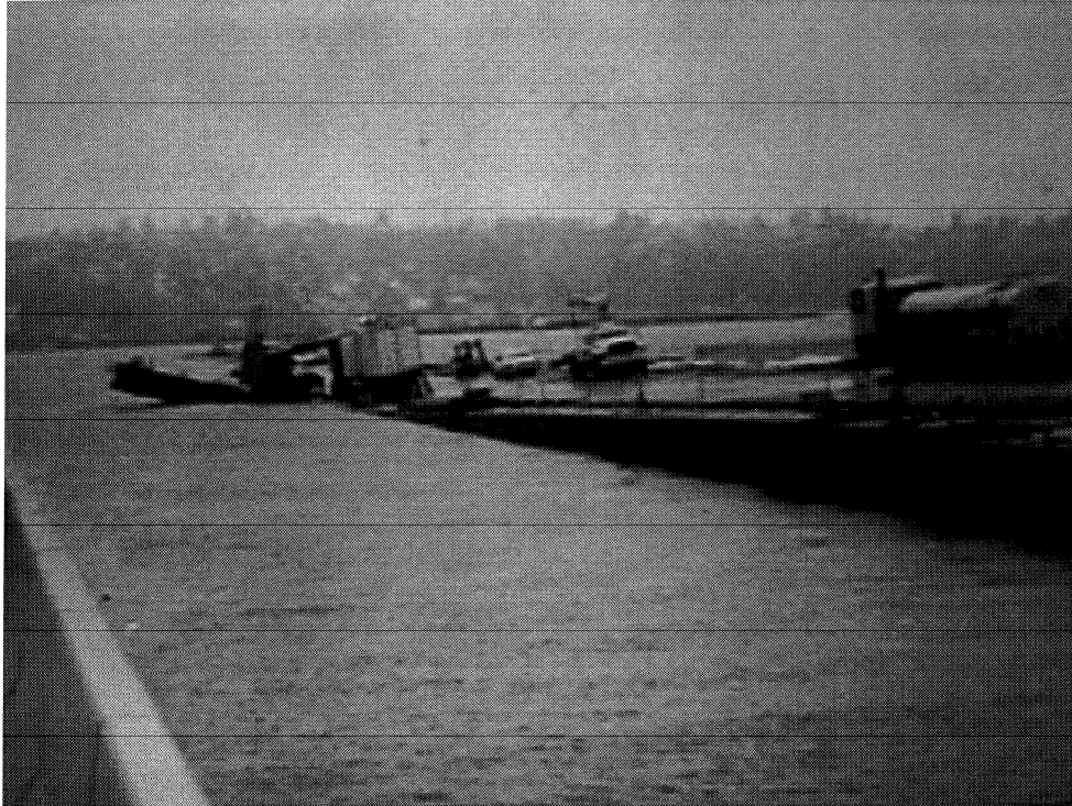
Photograph 3: Original Lacey V. Murrow Bridge sinking after a severe storm. 1990.
