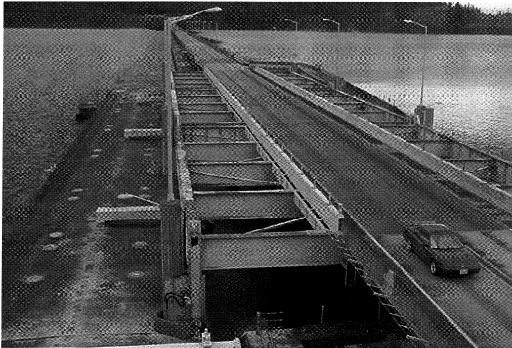
Photograph 12: Hydraulically operated lift spans at West half.
