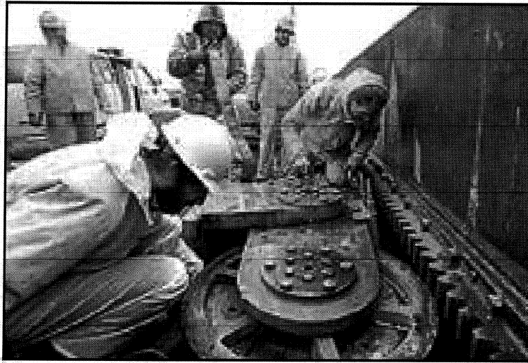
Photograph 22: Repairing damaged horizontal guide roller. 1999
