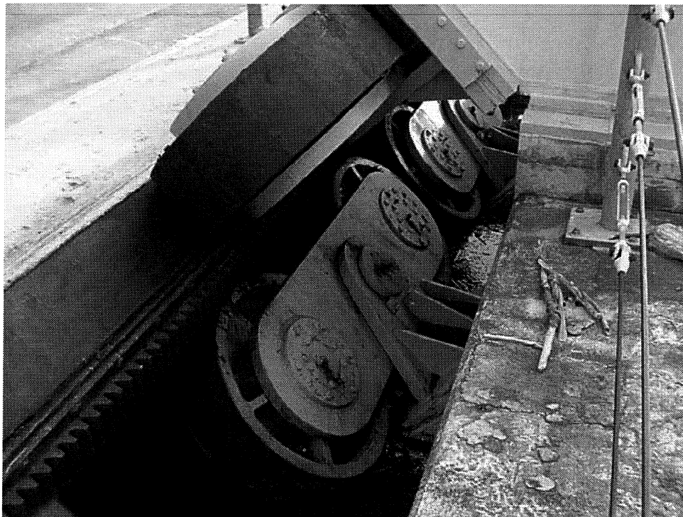
Photograph 19: West draw span guide rollers, guide track, and rack.
