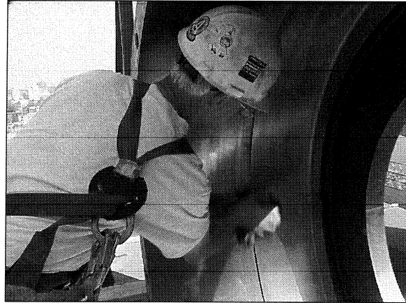
The bearing housing is being cleaned and prepped for bearing installation.
