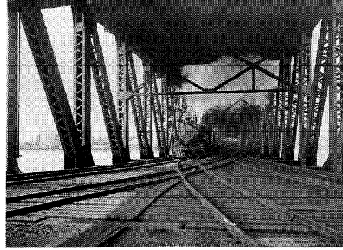
Steel Bridge carrying Rail Traffic on the Lower Deck (photo circa 1913) (collection of Hardesty & Hanover, LLP, New York)
