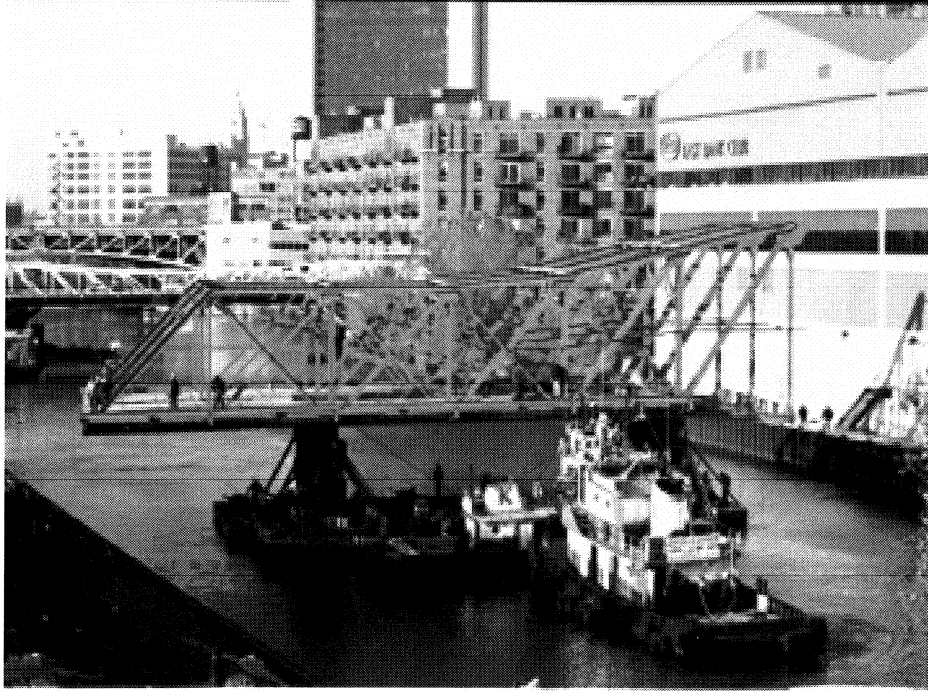
Kinzie Street Bridge Float-in of Trusswork
