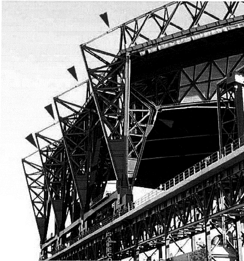
Figure 5 - Roof dampers on North side of truss
