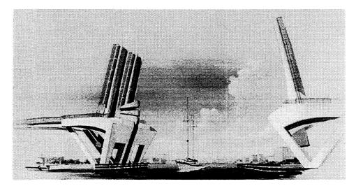
A major aesthetic goal of E.C. Driver was simple and clean lines. This philosophy is seen in the V shaped "Carina" bascule piers, and in the design of the bascule leaves themselves. Framing for the leaves consists of open box girders and floor beams. The inherent efficiency of the Exodermic design allows it to span the 14.4 feet (4.4 meters) between floor beams without stringers. Thus the underside appearance of the leaf, seen numerous times per day, is clean and uncluttered.
