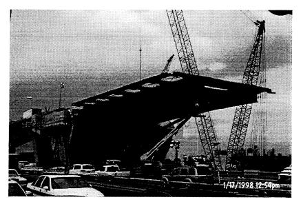
The new structure consists of long, segmental concrete approaches to twin, double leaf bascule bridges. Each double leaf bascule bridge spans 210 feet (64 meters) between trunnions, and is 53.5 feet (16.3 meters) wide. The first of the bridges opened for traffic in the spring of 2000.
