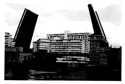
Engineers at consultant Reynolds, Smith and Hills evaluated bascule leaf designs with reinforced concrete, half-filled grid, and Exodermic decks. An Exodermic deck was chosen because it provided the lowest cost option for the overall design. By not requiring stringers, and by making the deck composite with the main girders and floor beams, using an Exodermic deck saved a substantial amount of structural steel. In addition, by not
