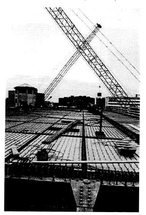
The main bars of the Exodermic deck are oriented in the direction of traffic, parallel to the main girders, and are made continuous over the floor beams through a bolted splice detail. Reinforcing steel in the Exodermic is continuous across the bridge in both directions, with standard lap splices as required. Main bearing bars of the deck are  $5^{3}/_{16}$ "
