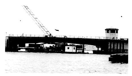
Parsons Brinckerhoff Quade & Douglas (PBQD) designed the replacement bridge, which is 171 ft. (52 meters) centerline pinion to centerline pinion. Main bascule girders are plate girders, 57'9" (17.6 meters) apart. Floor beams frame into the main girders, the top flanges of which are above the top of the finished roadway, at the level of the raised sidewalks. Floor beams are spaced at 13.5 foot (4.1 meter) centers.
