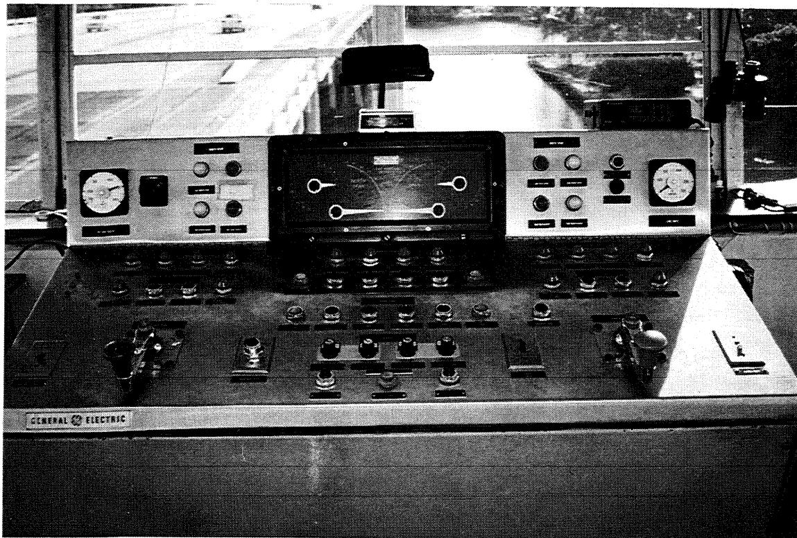
BEFORE: Existing Control Desk Layout (Drum Switches)
