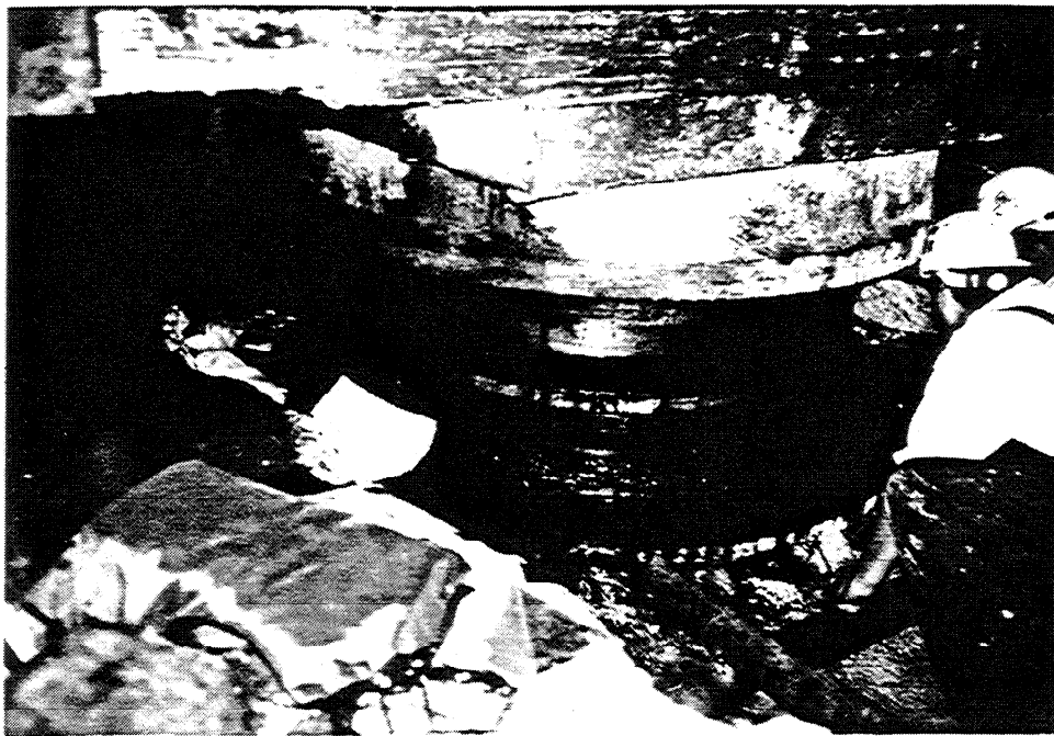
Photo 5 - Half of oil box removed. Note the high level of contamination found inside. Also note that the top steel lens was "stuck" to the upper pivot casting.
