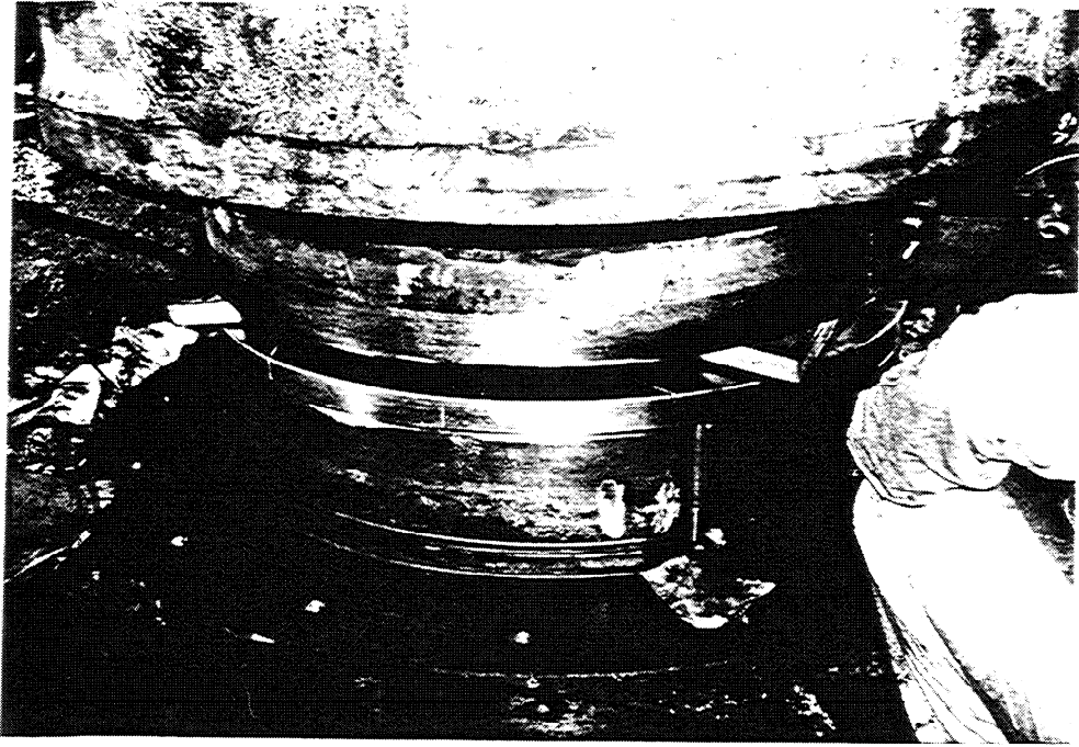
Photo 11 - Top steel lens being seated in the upper pivot casting.
