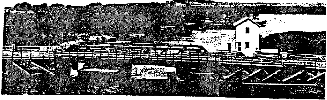
TYPICAL PONTOON BRIDGE, BUILT 1840 TO 1847. (Chicago Historical Society.)
