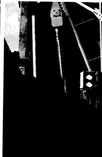
Heavy duty hydraulic cylinder; bridge in partially open position (2 cylinder/side)
