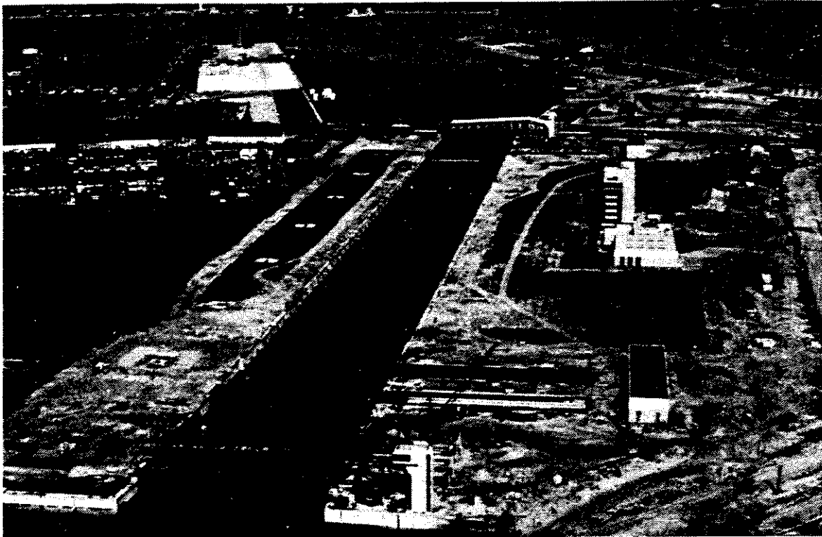
Fig. 17: Port of Zeebrugge, bascule bridges during construction (1980)
