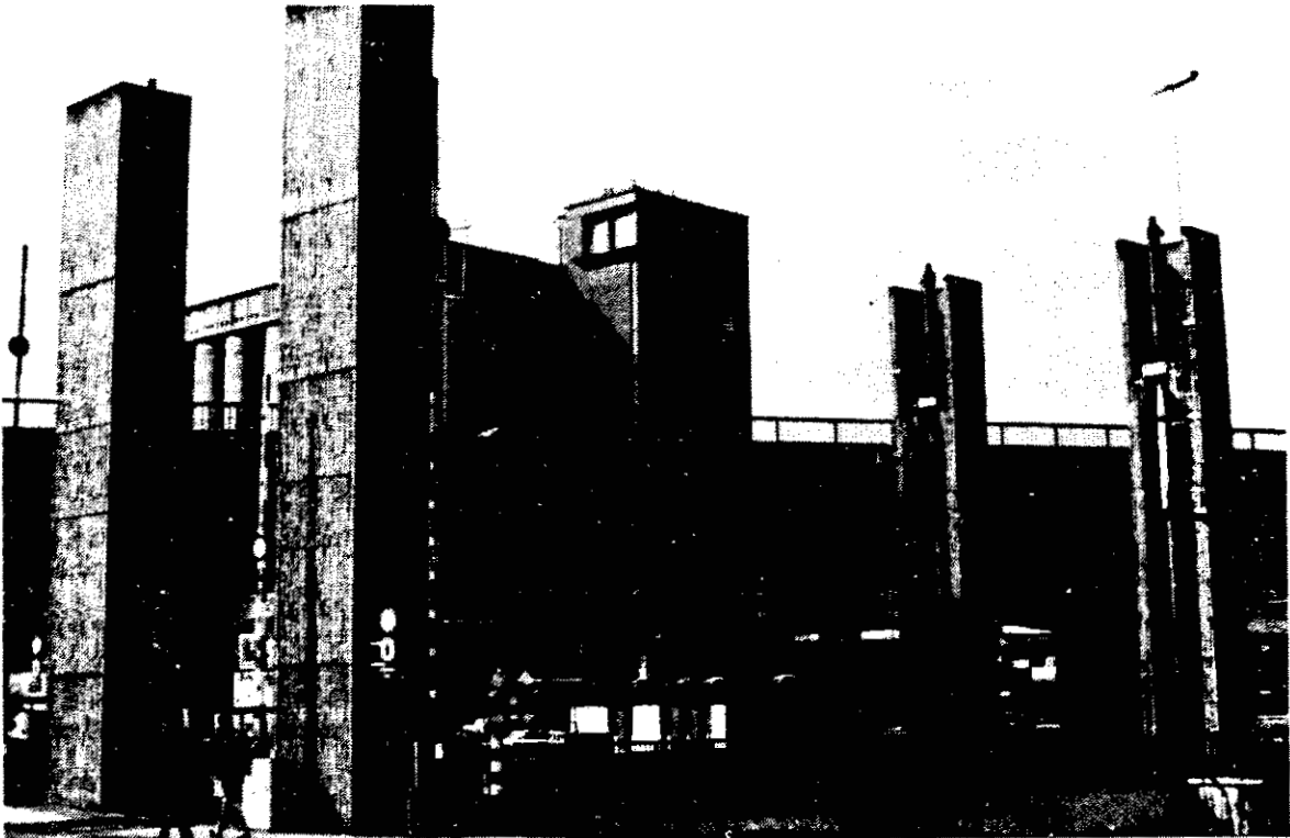
Fig. 21: Leuven, lift bridge without counterweight (1974)
