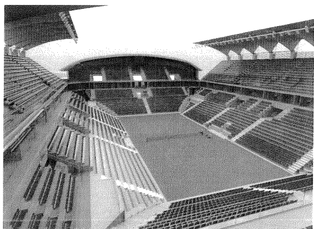
Interior view – roof opened, additional seating
